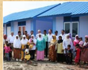
A community in Indonesia gathers with American Red Cross staff to celebrate the handover of their new homes. The American Red Cross and its partners supported the construction of more than 1,600 houses in Indonesia.
