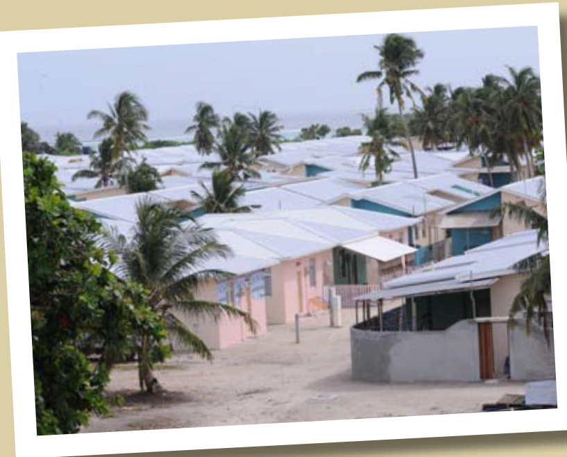
The American Red Cross supported the construction of houses, schools, community buildings, a municipal sanitation system and power supply facility on Dhuvaafaru, Maldives.
