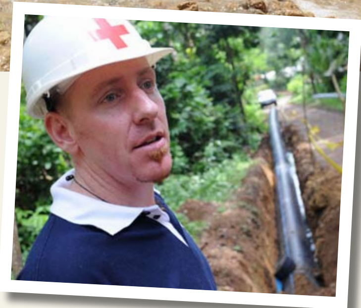
TOP: Boys play in water that has travelled through a 20-mile pipeline built by the American Red Cross in Calang, Indonesia. ABOVE: Kelvin Shingles, an American Red Cross water and sanitation delegate, explains how this pipeline will bring water to thousands of people in Galle, Sri Lanka, where many resettlement houses have been constructed.
