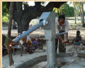
The water source pictured here is one of many provided by the Red Cross in coastal areas of Kenya. This project, which benefited 45,000 people, also improved sanitation systems and taught hygiene promotion.
